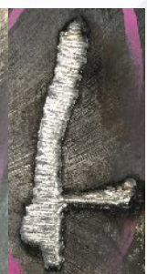
FC230 crack repair.
